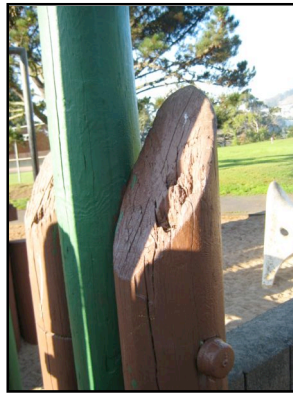
Deteriorating wood
